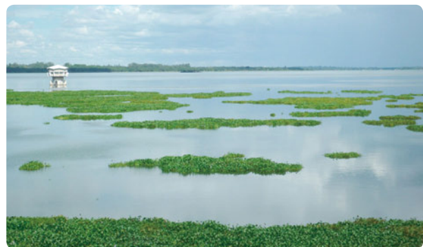
Lake Chivero water intake infested with water weeds
