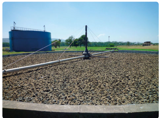
A seriously dysfunctional sewage treatment plant under partial repair
