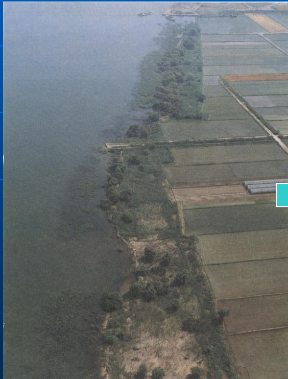
Before dike construction
